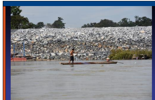
Don Sahong Coffer Dam
